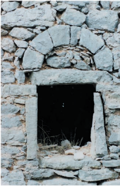
Picture 10. Foundation on the rock
