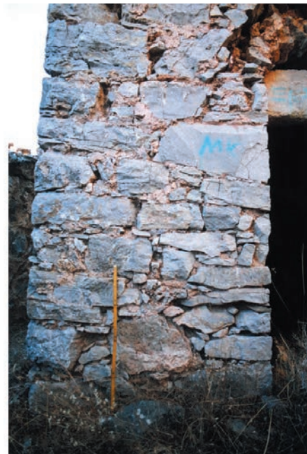
Picture 9. Interior of the building
