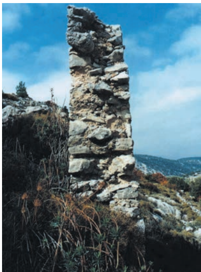
Picture 4. Masonry structure
