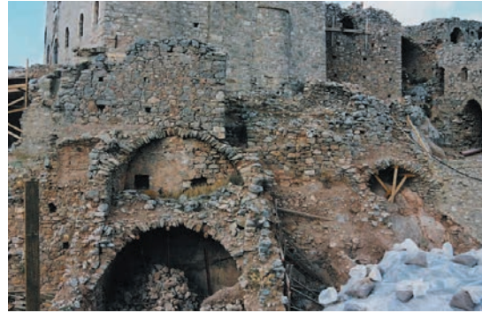
Picture 7. Construction of successive domes.
