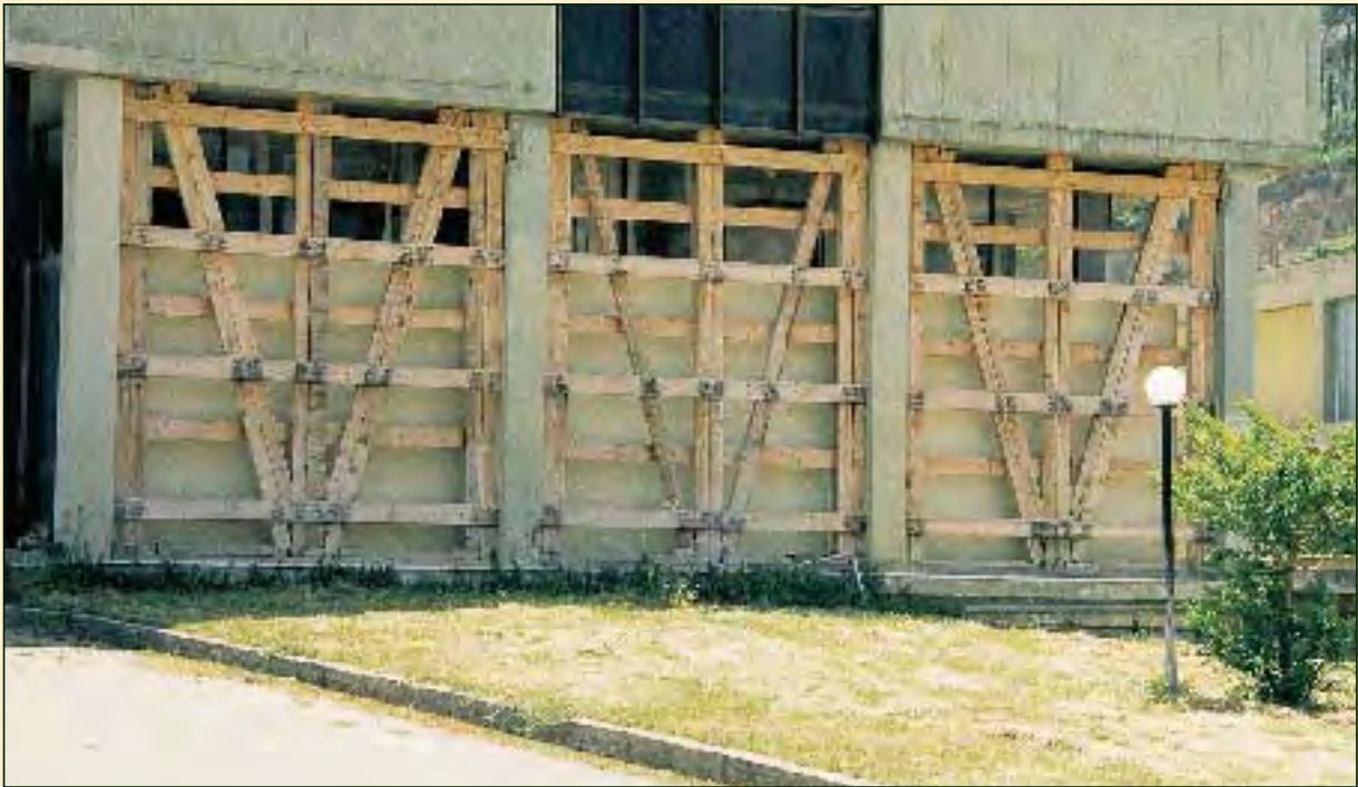
Egion 1995 Perimetric shoring with timber.
