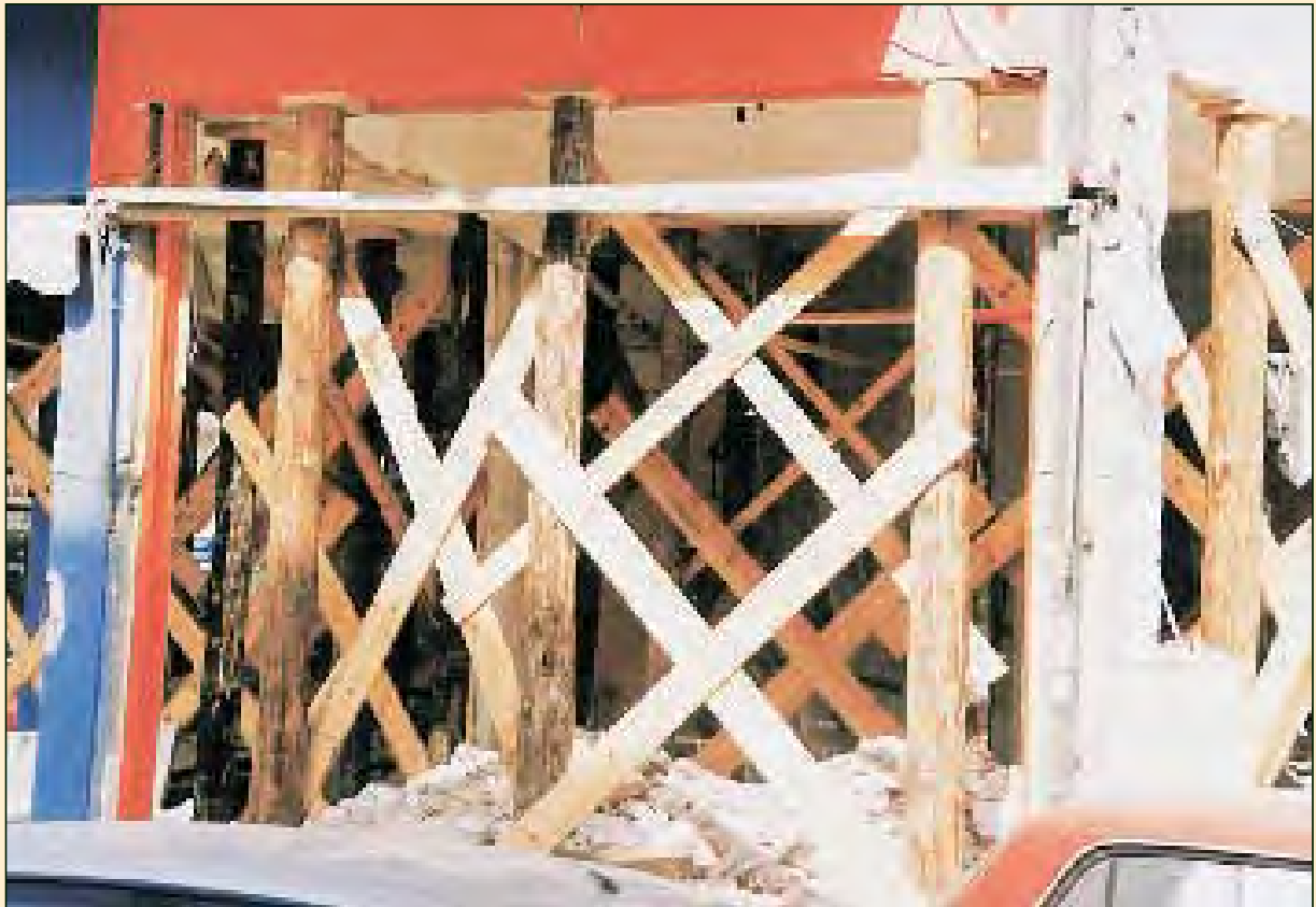
Attika Ano Liosia 1999 Propping with tree trunks.
