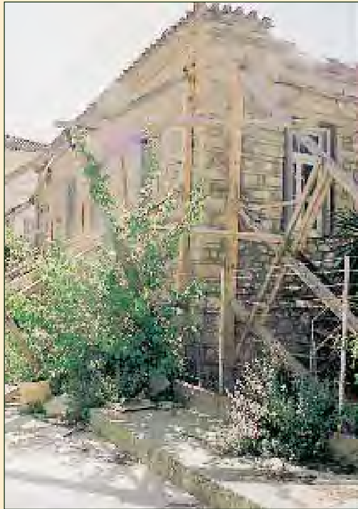
Egion 1995 Shoring using industrial timber
