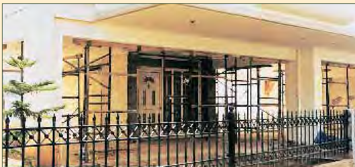
Attika – New Herakleio 1999 Extended propping using whole sections in pilotis with heavy damages on many columns.
