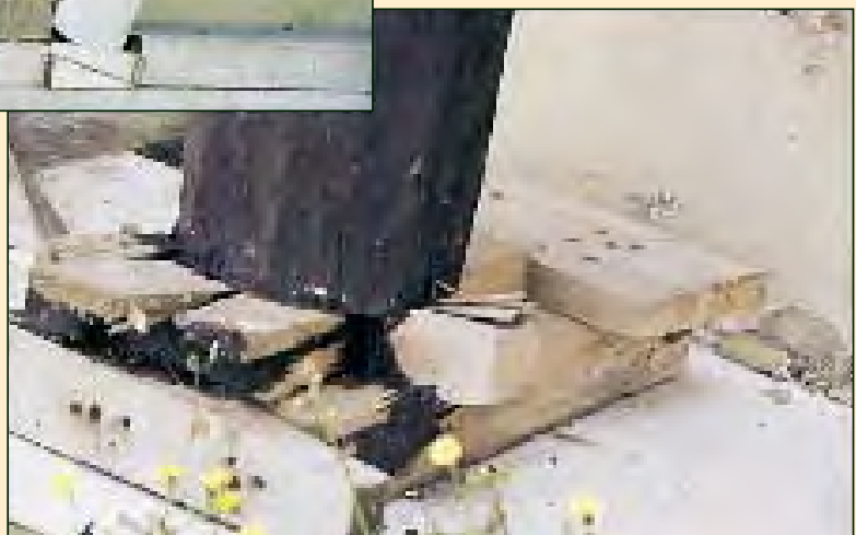
Wrong wedging on tree trunk propping.
