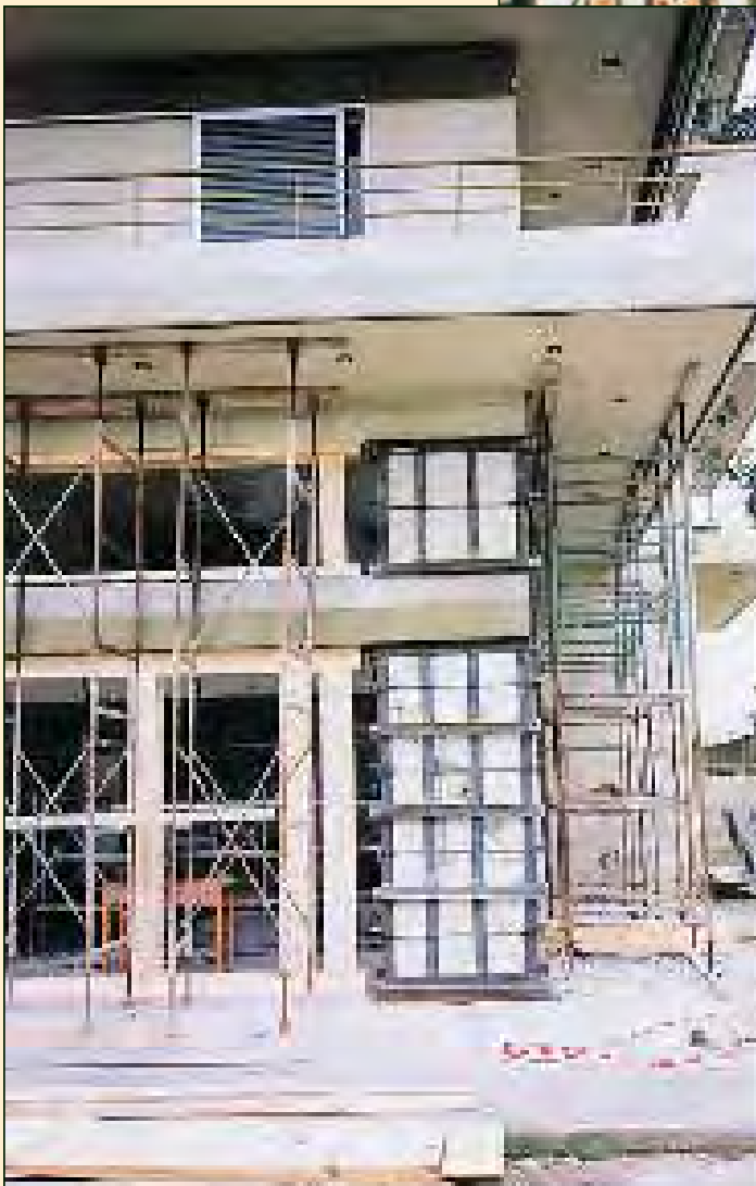
Pyrgos 1993 Propping using tightening procedure
