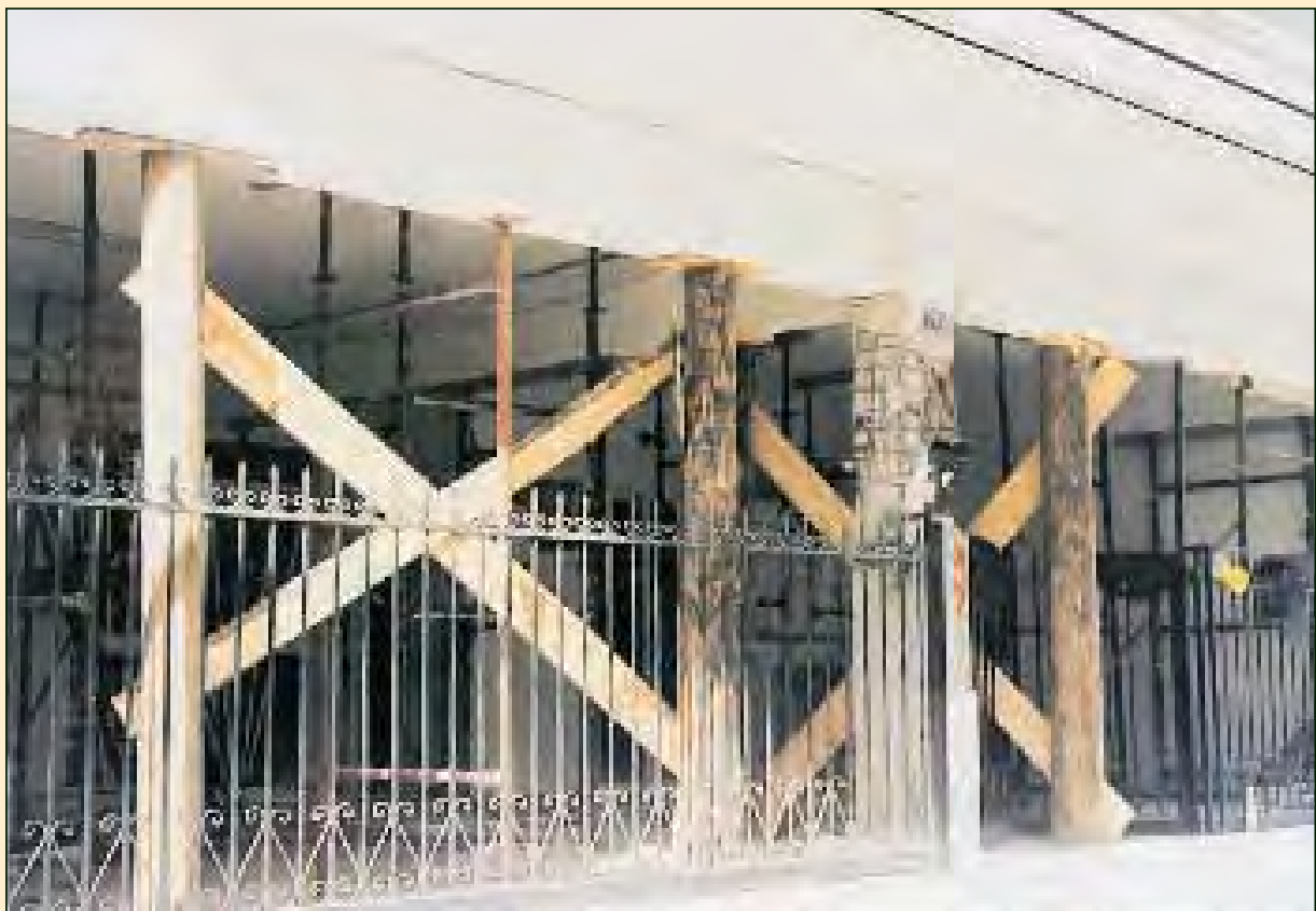
Attika – Ano Liosia 1999 Propping using tree trunks
