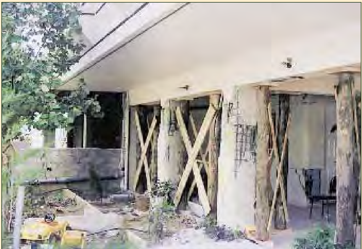
Attika Ano Liosia 1999 Propping with tree trunks.
