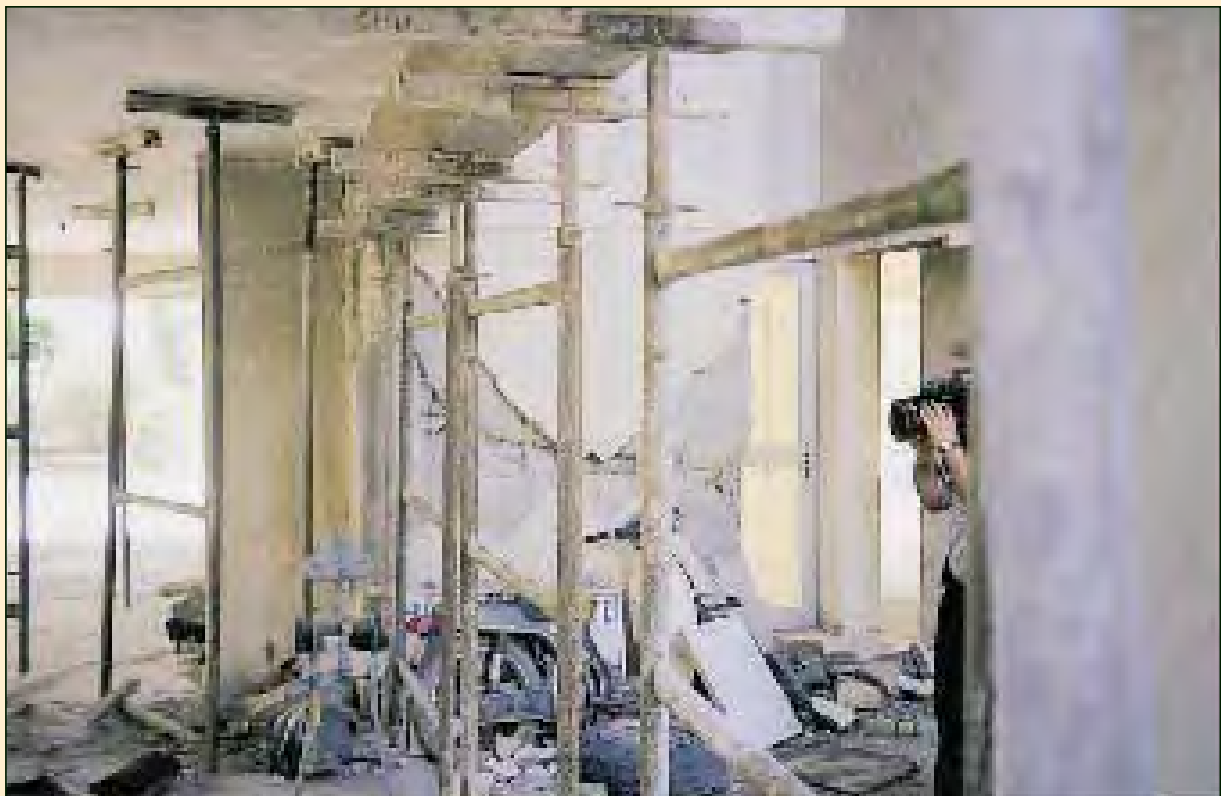
Paphos – Cyprus 1995 Temporary dense propping with metal scaffolding.
