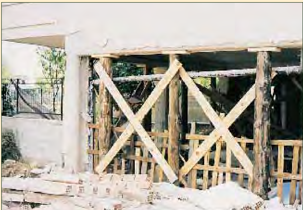
Attika – Ano Liosia 1999 Propping using tree trunks
