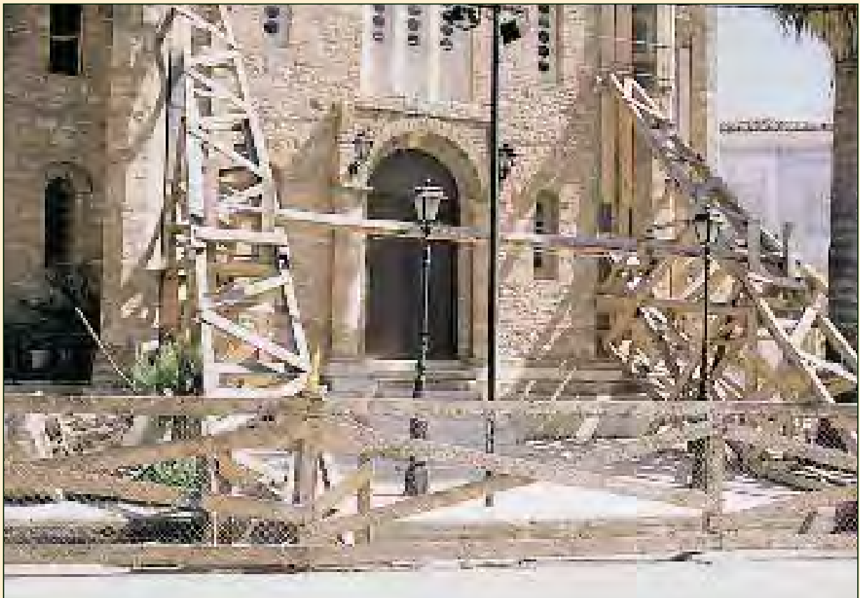
Egion 1995 Extended shoring using industrial timber on a traditional church bilt by Chiller .
