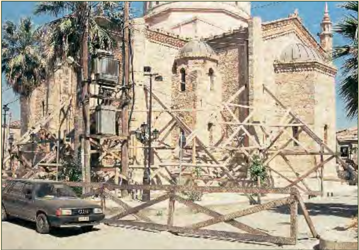
Egion 1995 Extended shoring using industrial timber on a traditional church bilt by Chiller .
