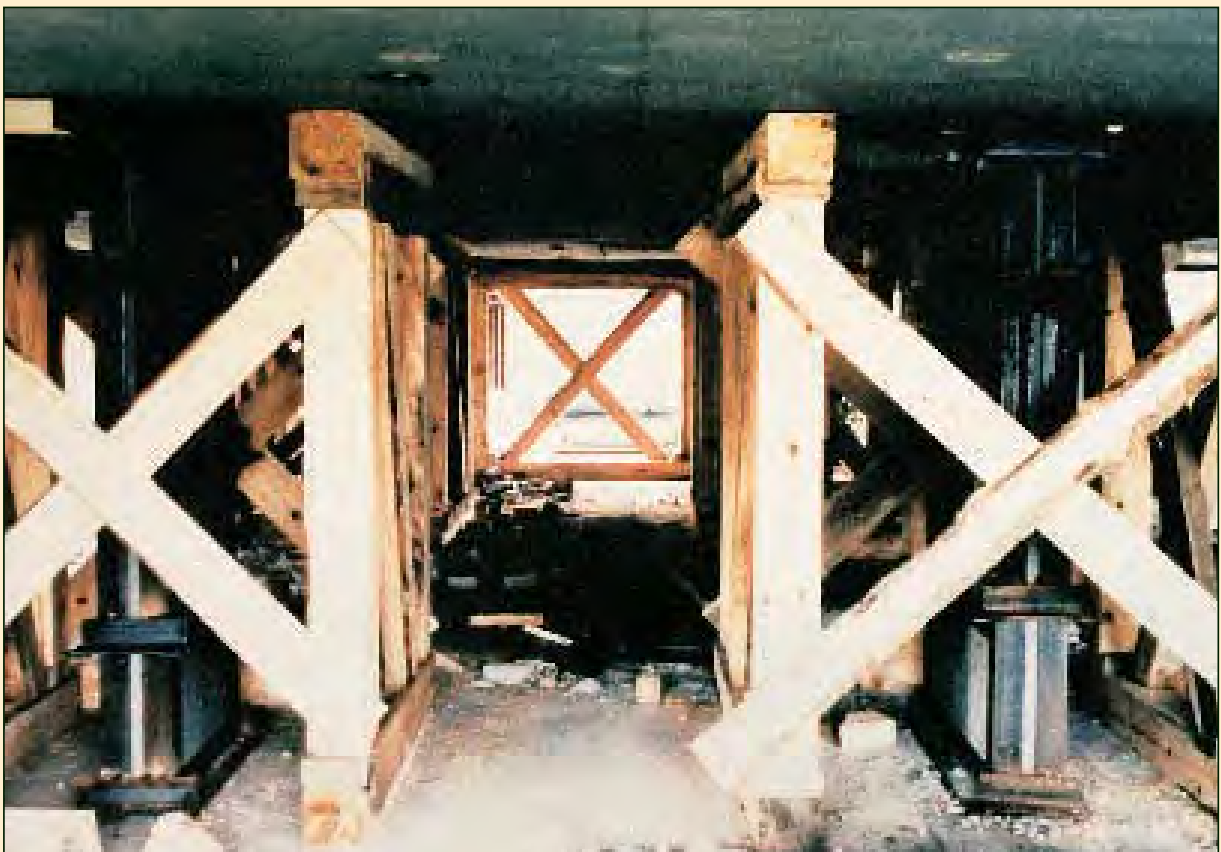
Kalamata 1986 Propping – shoring with industrial timber and tightening with metal angular elements on all damaged pilotis columns
