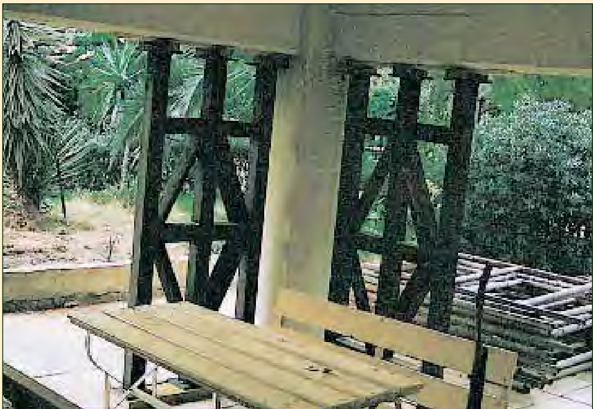
Attika – New Herakleio 1999 Extended propping using whole sections in pilotis with heavy damages on many columns.
