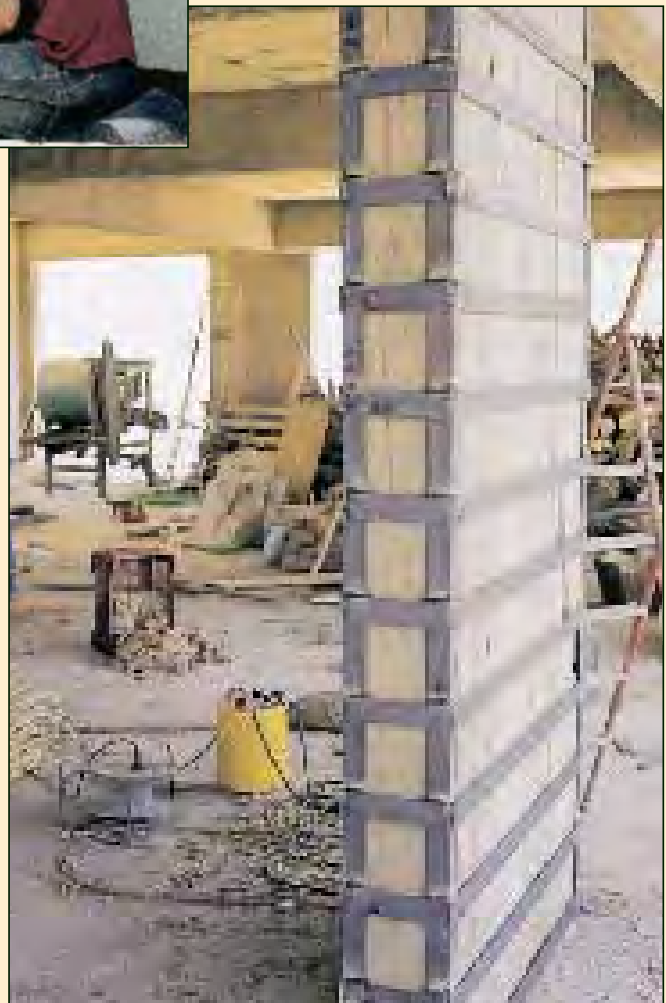
Egion 1995. Tightening using metal plates.
