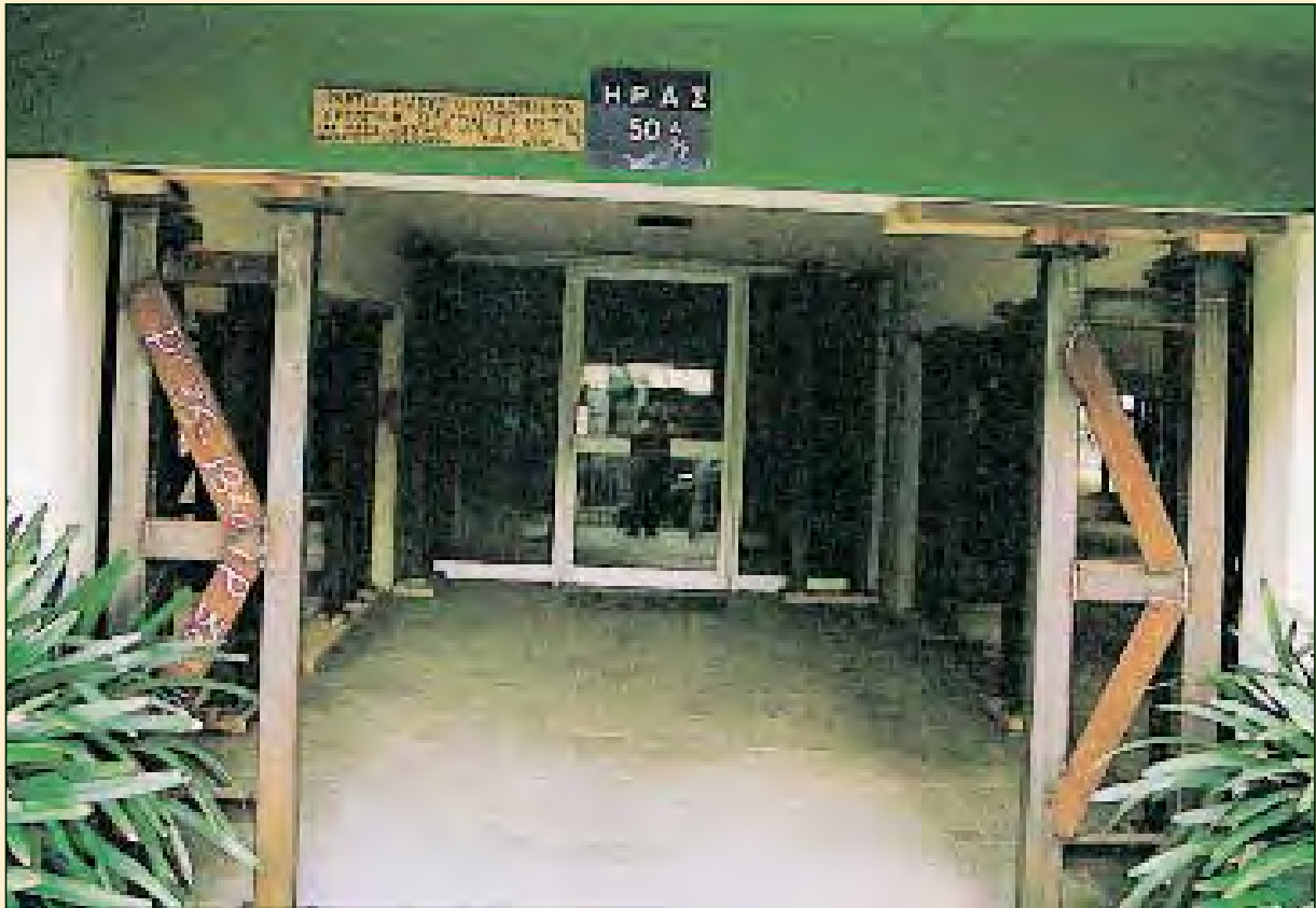
Attika – New Herakleio 1999 Extended propping using whole sections in pilotis with heavy damages on many columns.
