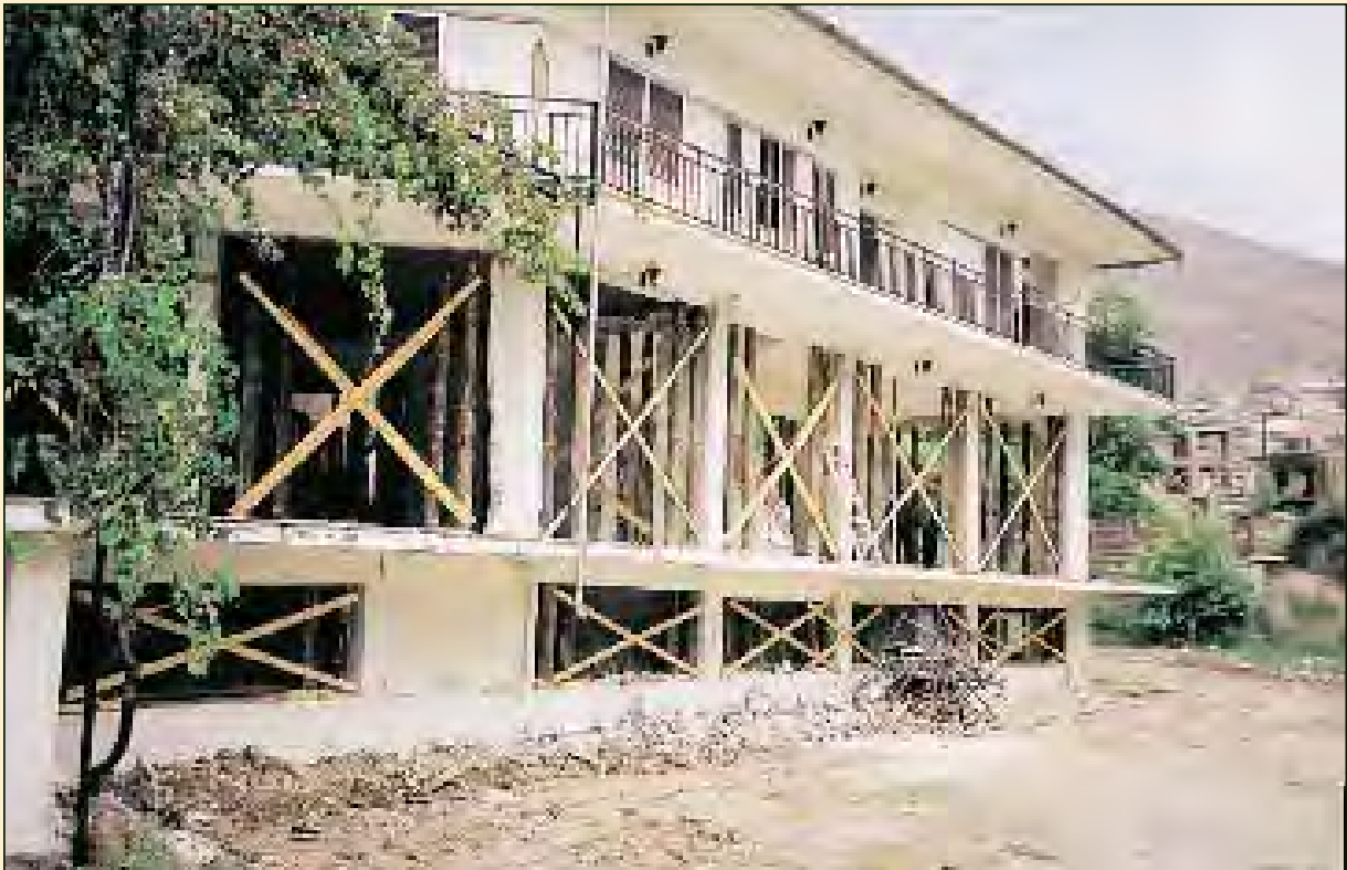
Extended propping using tree trunks. The propping has been applied on the ground floor and basement.
