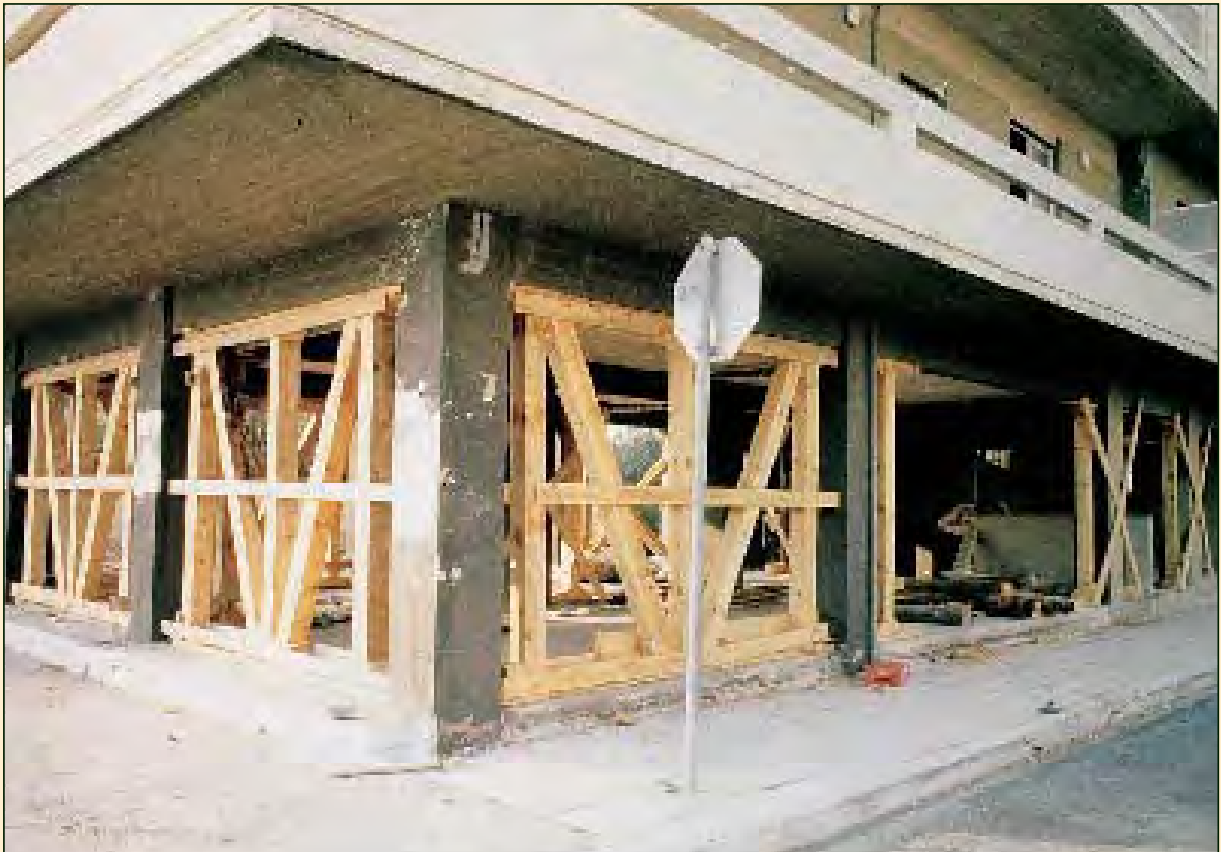
Kalamata 1986 Propping – shoring with industrial timber and tightening with metal angular elements on all damaged pilotis columns
