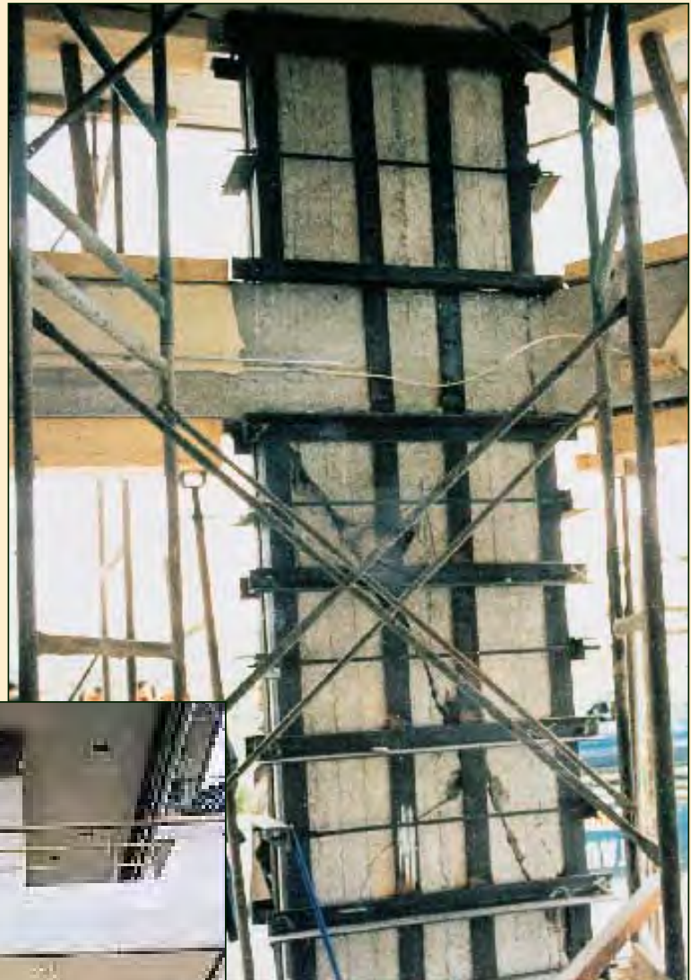
Pyrgos 1993 Propping using tightening procedure
