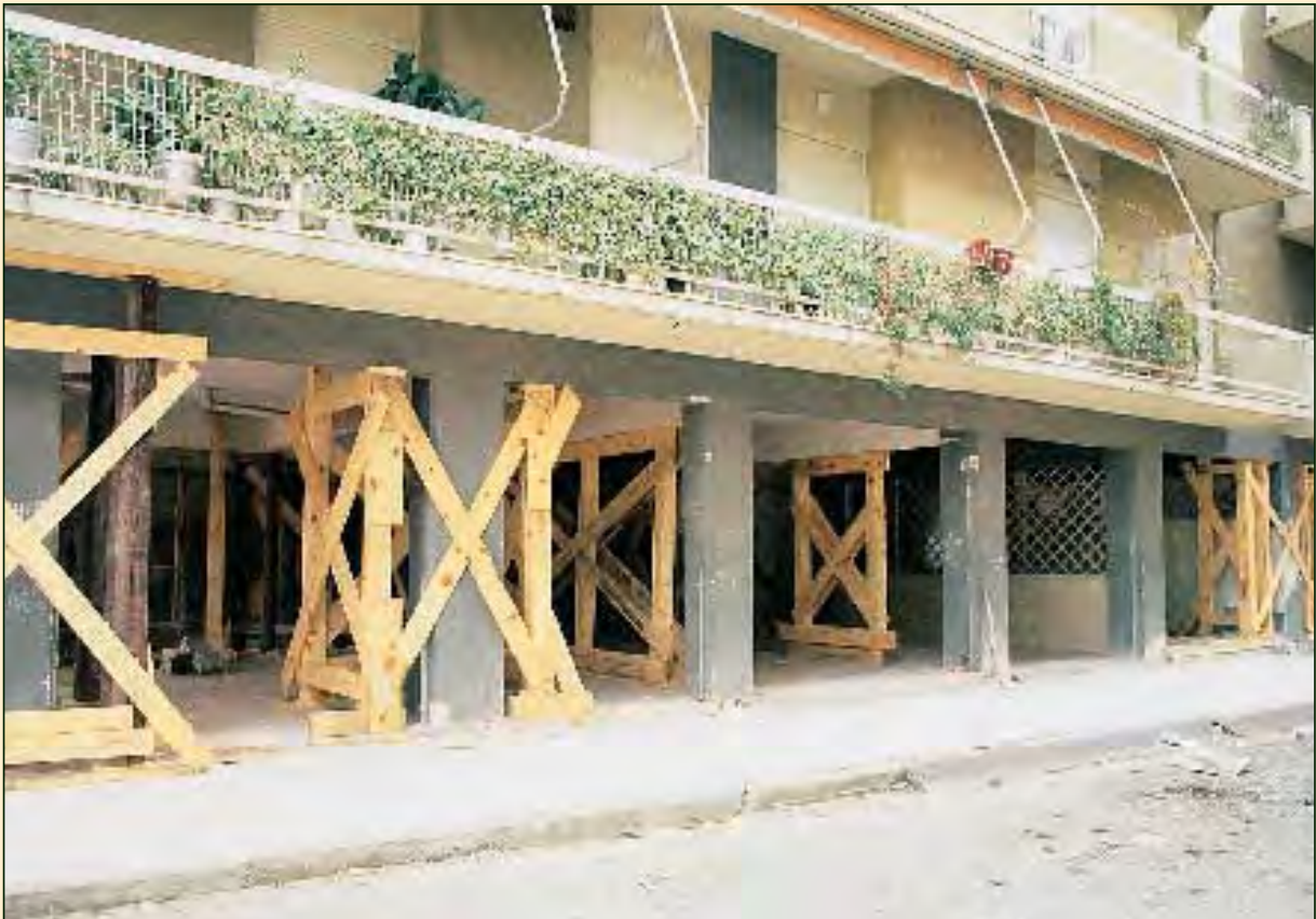
Kalamata 1986 Propping – shoring using industrial timber
