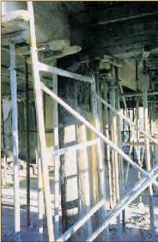
Paphos – Cyprus 1995 Temporary dense propping with metal scaffolding.
