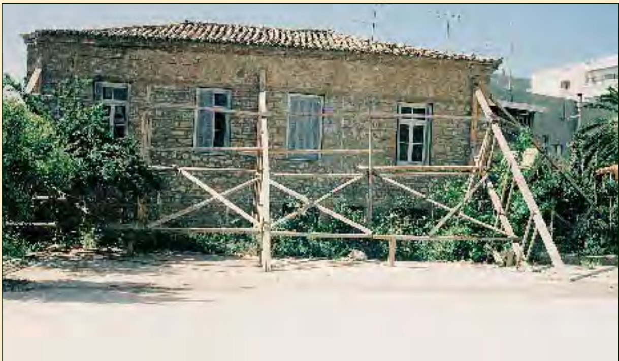
Egion 1995 Shoring using industrial timber
