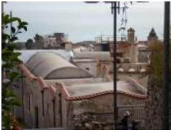
Photo 1: Ravello - Example of extradosed vaults
