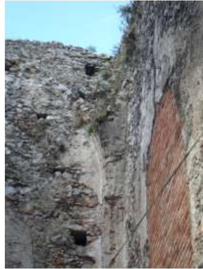
Photo 4 Ravello - The beginning point of a vault
